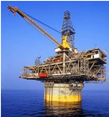
Figure 1 – Spar Dry Tree Production Facility, Reference 3
