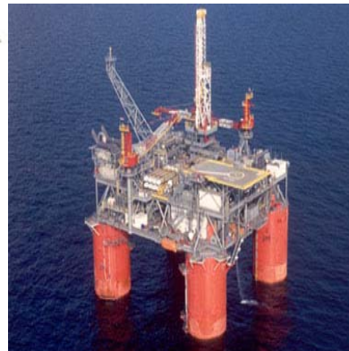
Figure 2 – TLP Dry Tree Production Facility, Reference 6
