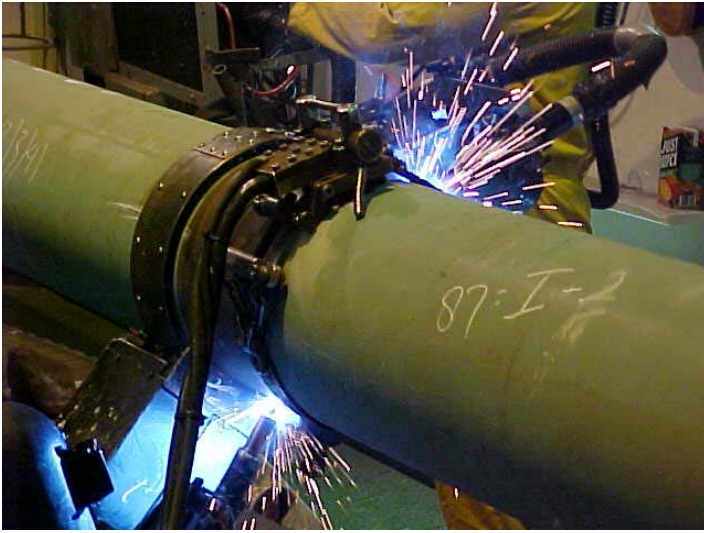
Figure 8 – Automatic GMAW Welding of the West Seno Export SCR
