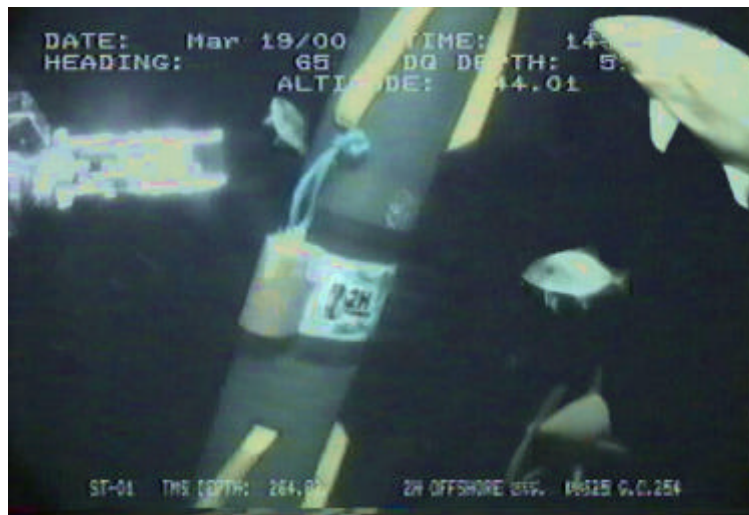
Figure 10 - 2H Accelerometer on the Allegheny SCR
