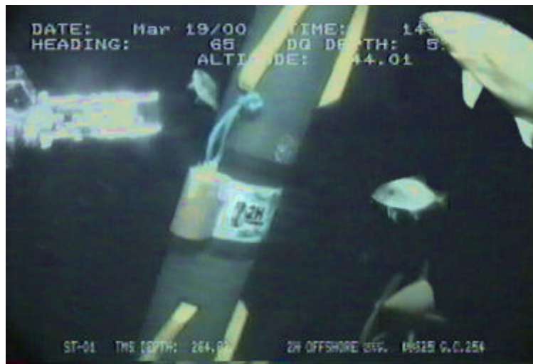
Figure 2 - 2H Accelerometer on the Allegheny SCR
