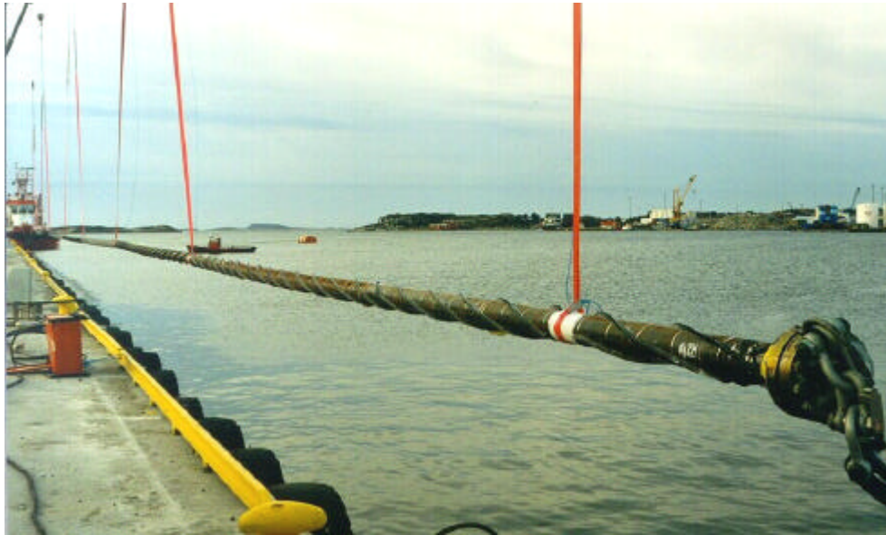
Figure 1.3 – Lifting out the Straked Pipe
