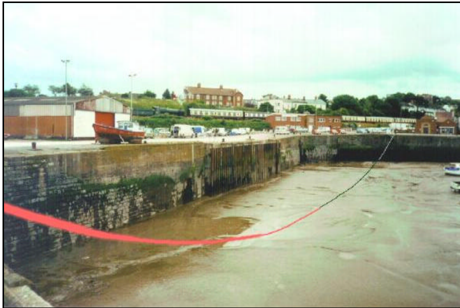
Figure 1.7 – Harbour TDP Tests (modified photograph)
