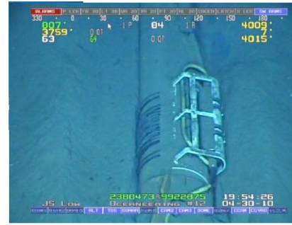
Figure 2: Monitoring device located at SCR touch down zone.
